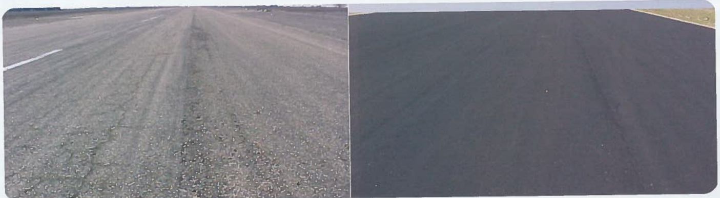
As shown in the photo on the left, the Abernathy Municipal Airport runway was in poor condition with multiple pavement failures. The photo on the right shows the improved runway immediately after a slurry seal.
