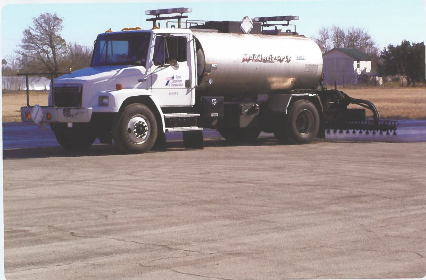
RAMP in action: A fog seal is applied to the runway at Wills Point Municipal airport.
