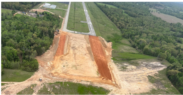
Construction under way at Wood County Airport Collins Field runway 18-36.
