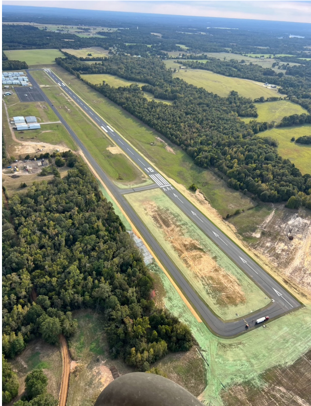
Completed construction on runway 18-36.
