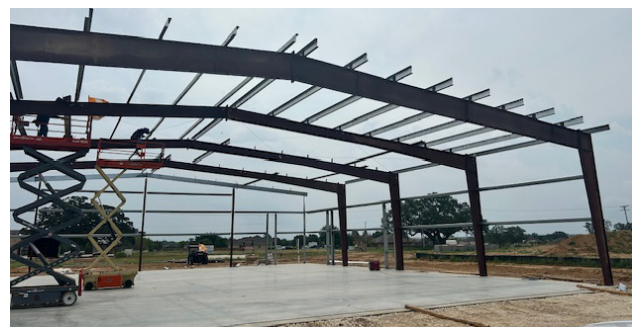
New hangar under construction at Pleasanton Municipal Airport.
